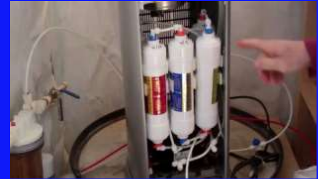
TAP WATER REPAIRING
